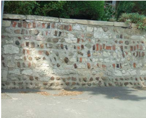
Stone wall with brick and cobble infill and stone coping.
