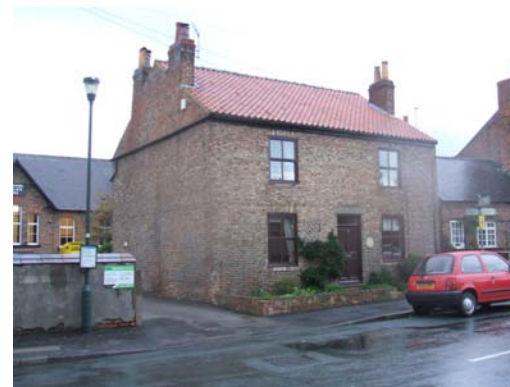
Chimney stacks with the thickness of the wall.
