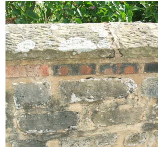
Stone wall with brick lacing lcourse and stone coping.
