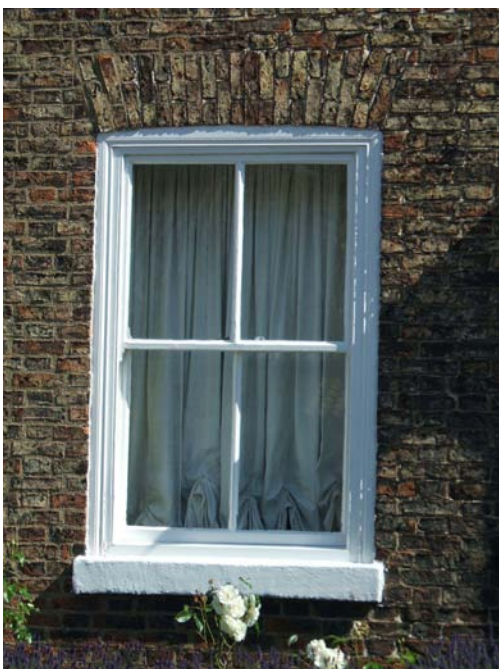
Vertical sliding sash window.
