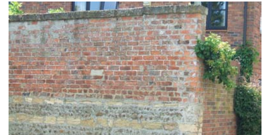
An important boundary wall now included in the Conservation Area.
